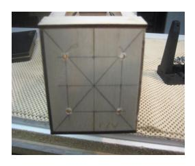
\*Position and glue in place the bottom I/s reinf. Front.
