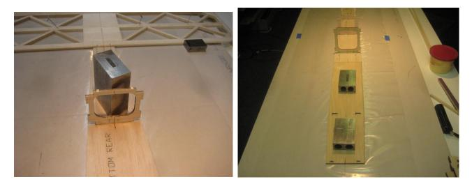
\*Prepare former #2 by gluing two 1/8" laser cut plywood #2 formers together holding the periphery of the parts flush and lining up the 1/4" dia holes.
